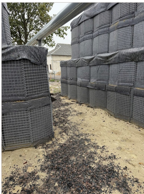
Filled HDGDEF units with geotextile lining
